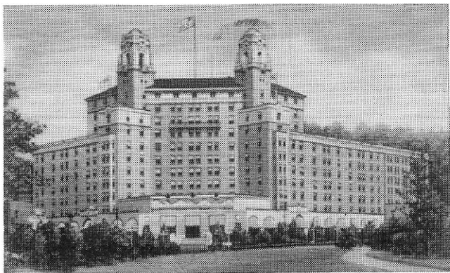
The New Arlington Hotel in Hot Springs, the original location of radio station KTHS.
