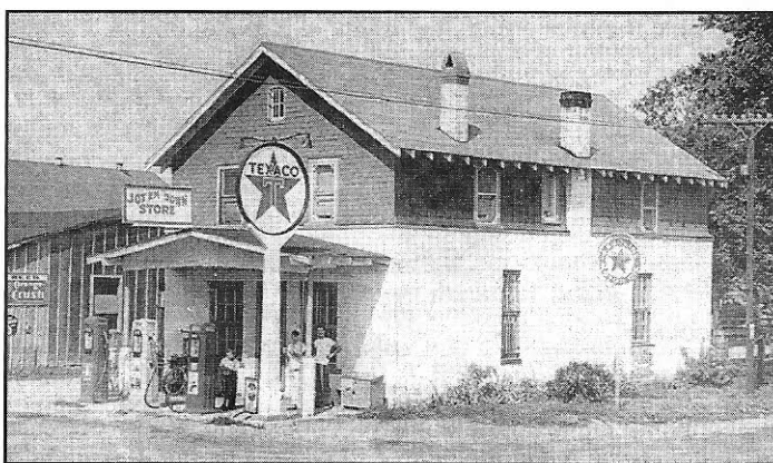
The Lexington, KY, "Jot 'Em Down Store" as it appeared in 1943. Notice the hanging sign, which was personally commissioned by Lauck & Goff.
