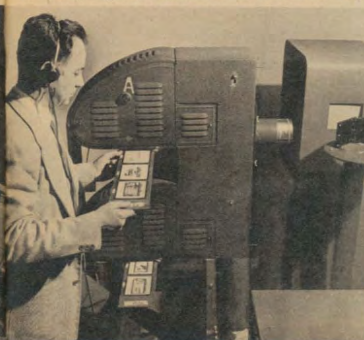
In the CBS studio, an engineer inserts slides advertising Ford's wares into a balopticon projector during time-out periods. Ford also uses movie shorts as commercials.
