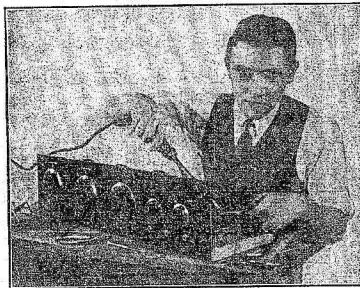
Front View KD-50, Neutrodyne Being Assembled
