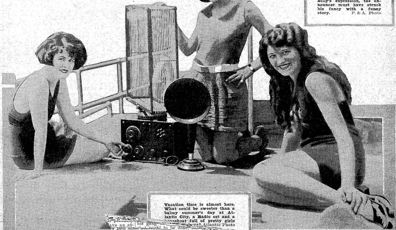
A two-tube reflex has been installed in an old phonograph cabinet, by an ardent Philadelphia Radiophan. Everything has been removed from the case but the horn, and that is connected direct to the set. ©Keystone
