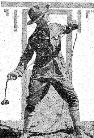
Portable set aeriels are easy enough to erect—if one knows how. Here a Boy Scout has volunteered to demonstrate. Tie a weight to the end of a fifty-foot length of single lamp cord, and toss the end over a convenient bough.
