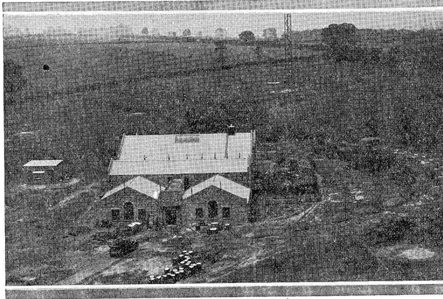
Looking down from an airplane on the power house of the new superpower station, 5XX, at Daventry, England, the gigantic proportions of the equipment can be visualized. The broadcaster recently was opened and now is an important link in the British Broadcasting company's scheme. 5XX operates with 25 kilowatts (25,000 watts) of power on a wave length of 1,600 meters. The above photo was presented to Fred Smith of WLW during his visit at Daventry.
