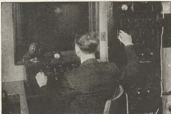
A portion of our broadcast studio control equipment
