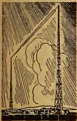
The towers of WLW. The transmitting unit of this station is located near Mason, Ohio—about twenty-five miles from the center of Cincinnati, far away from population congestion
