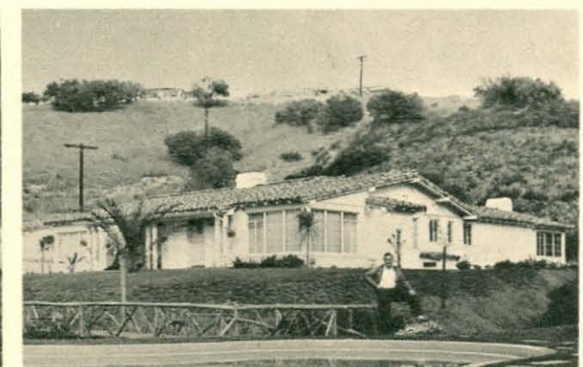
Adjoining Jolson estate is home of Phil Harris and his actress wife, Marcia Ralston. Windows in fore corner open from Phil's bedroom
