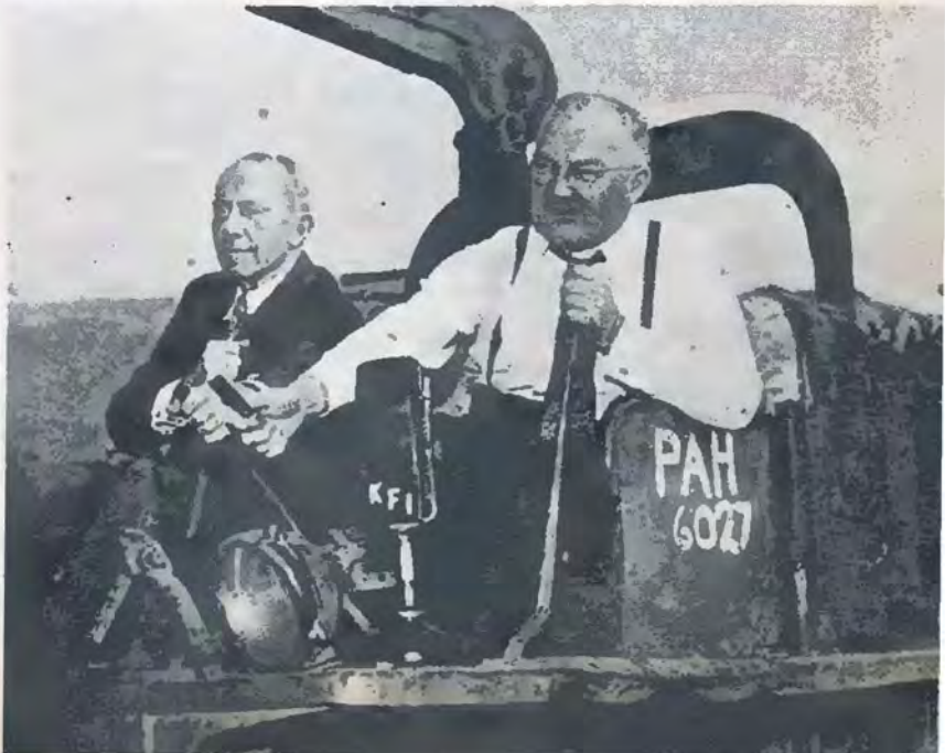
A WORKING MAYOR —Fletcher Bowron of Los Angeles is shown operating the bulldozer used to break ground at the site of KFI's new television and FM transmitter atop Mt. Wilson last November. The gentleman assisting is Eugene Overton, KFI's legal representative, who is also president of the city's board of harbor commissioners.
