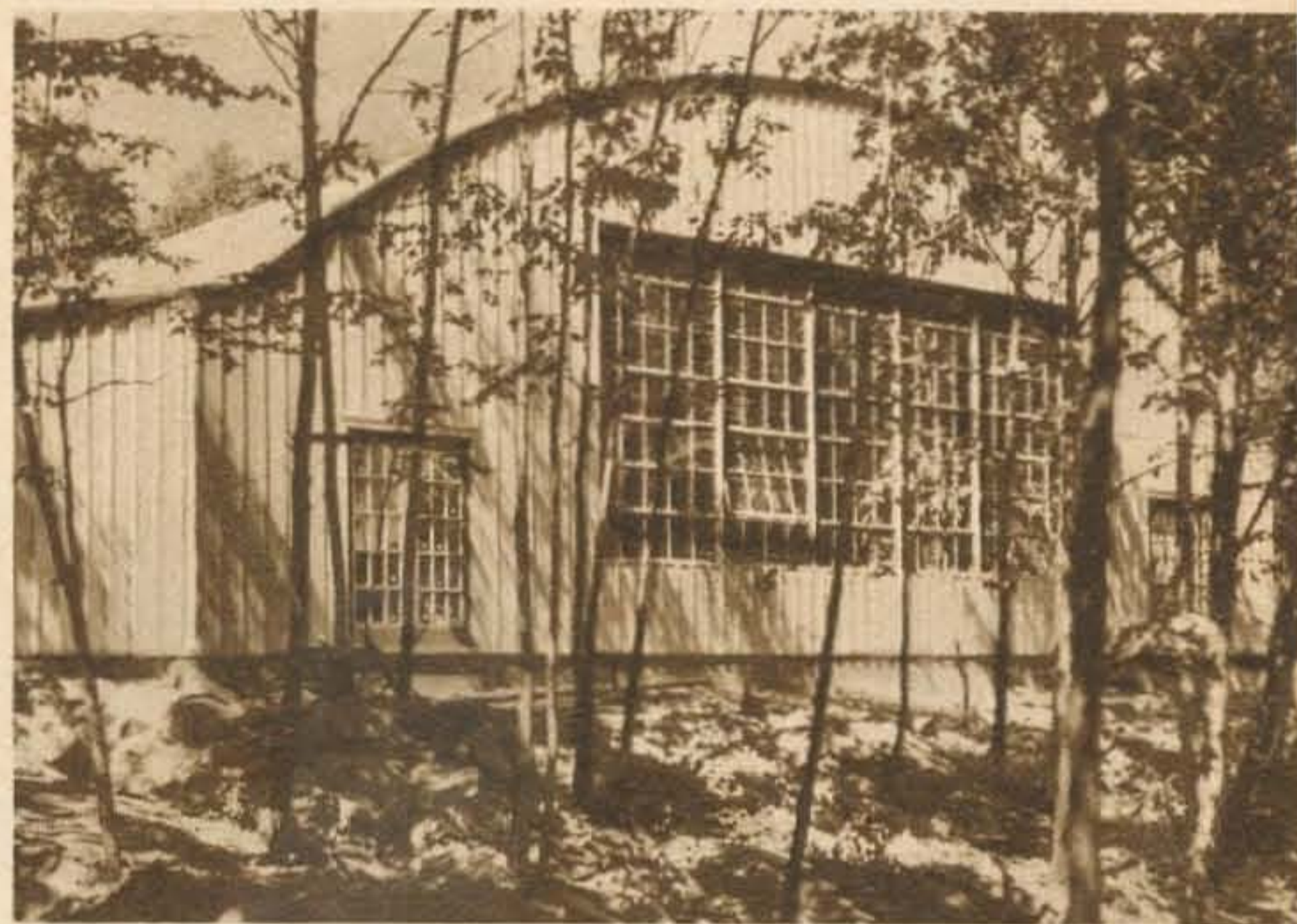
Also built by listeners' gifts is this pavilion, nearly completed, which will be used as a rest-house for the parties of pilgrims who frequently come to Graymoor.
