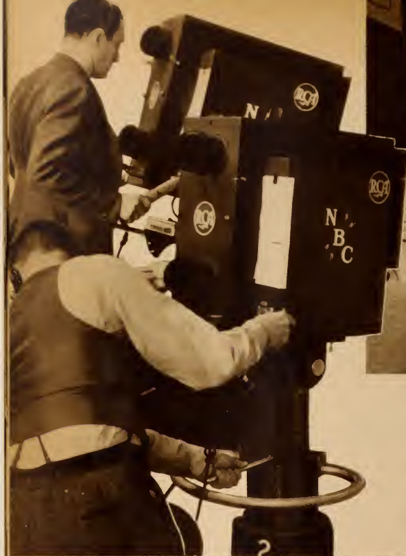
During the past year more than sixty television demonstrations have been given by NBC, who have spent vast sums pioneering in the field of program material and with the color response of facial make-up and costume fabrics. (Left) The Iconoscope (television camera) nearest you is used for close-ups. The other is mounted, so as to be moved forward or back. Make-up (above) is greatly simplified, due to changes in the Iconoscope. Lester Gabba (lowest left), artist and designer, introduced his mannequin, Cynthia, at NBC's All-Fashion Television demonstration, showing small accessories.
