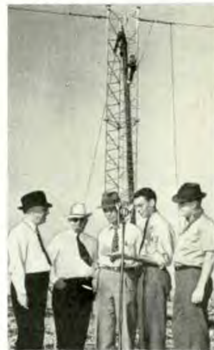
NEW WFAA TOWER
