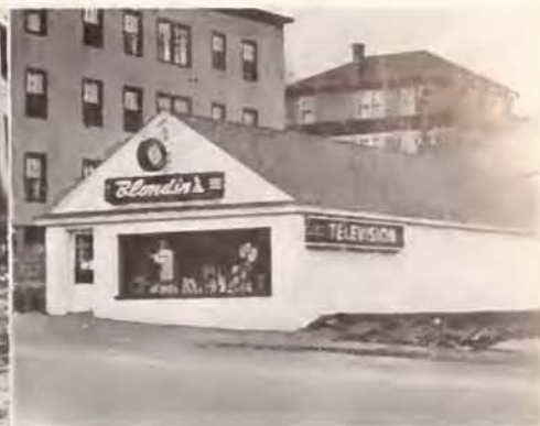
After: new buildings that radio helped build. Blondin's uses the air the year 'round
