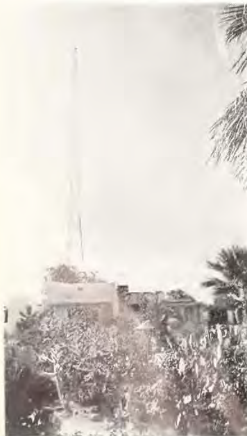
KOY transmitter property and single tower, giving non-directional coverage over 85% of Arizona's population with 5000 watts on 550 KC. A 5 KW main transmitter and 1 KW standby, with auxiliary power plant, are both Western Electric equipment of the latest design.
