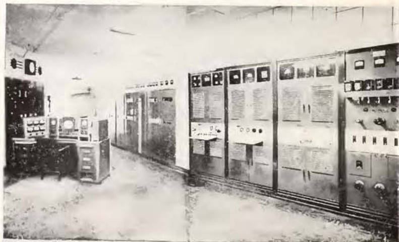
INTERIOR of WMBG transmitter building. WMBG now uses FM tower as radio AM signal, providing a very substantial increase in WMBG coverage of the State of Virginia.
