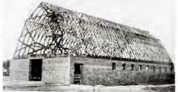
Blackburn College, famous "self-help" school at Carlinville, Illinois, needed a new barr. President Hudson, well known to network listeners as well as on individual stations, told the public. The bricks in the wall came from an old street pavement. The oak lumber was sawed on the college farm. Radio listeners helped with incidental expenses.
