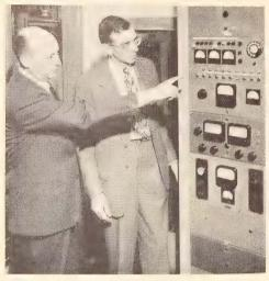
CHARLES DILLON (I), vice president-general manager of WOL Washington, D. C., and Henry Rau, president, examine a centralized control rack recently installed by Gates Radio Co. to provide a remote control system for the station's three transmitters. Two of the transmitters, a 10 kw fm and 50 w am booster, are at one location while the main 250 w am transmitter is at another.
