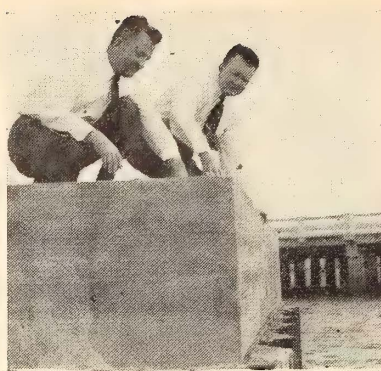
M. C. SCOTT (l), chief engineer, WIOD Miami, Fla., explains to J. Leonard Reinsch, managing director, Cox stations, details of the construction of a concrete anchor for one of the new hurricane-proof towers being built at WIOD's transmitter site in Biscayne Bay. Total weight of the concrete and steel in the three anchor foundations and the tower base foundation is 3,527,000 lbs.
