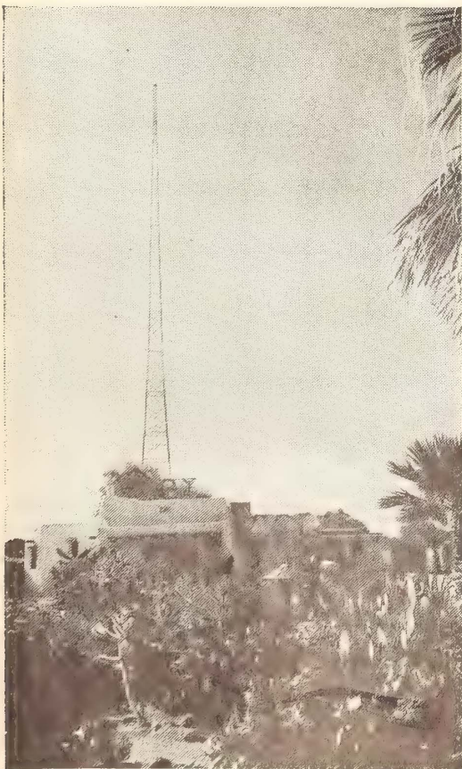
KOY transmitter property and single tower, giving non-directional coverage over 85% of Arizona's population with 5000 watts on 550 KC. A 5 KW main transmitter and 1 KW standby, with auxiliary power plant, are both Western Electric equipment of the latest design.
