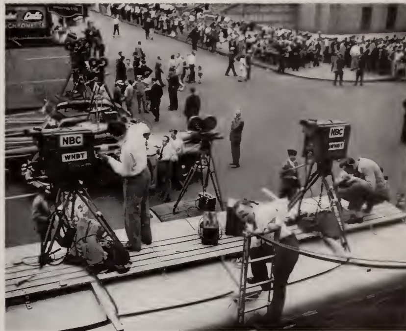
Checking cameras on top of truck before American Legion Parade. Coaxial cable is strung alongside the ladder.
