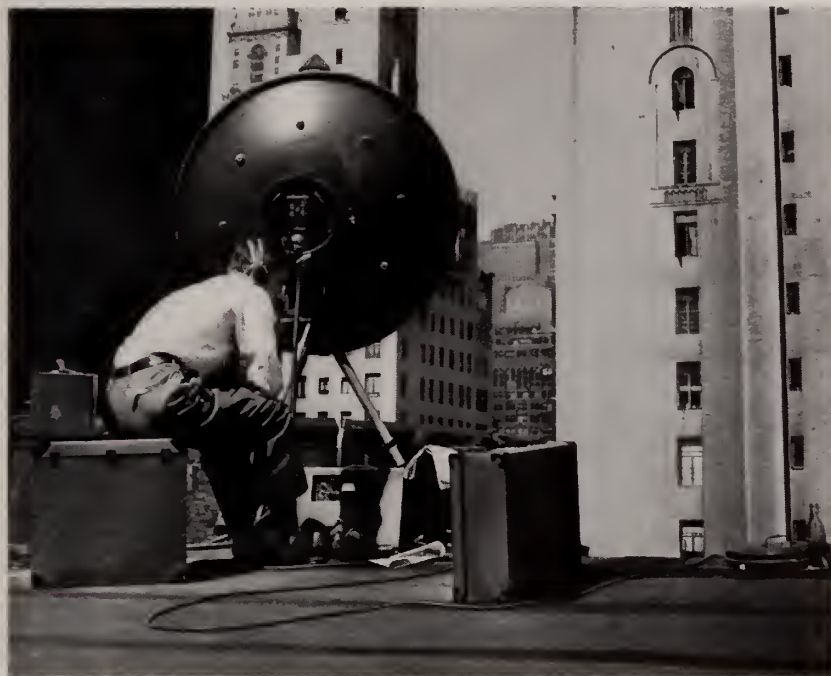
Parabolic transmitter, popularly called the "dish," reflects microwaves to the RCA Building in the distance.
