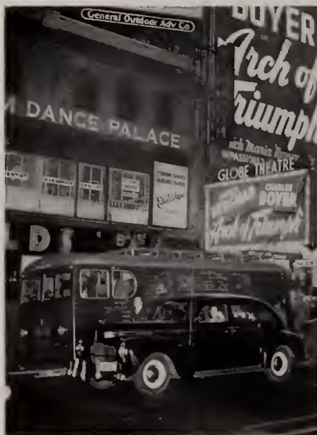
NBC Television attends the Arch of Triumph premiere. Power cables are strung from the marquee to the truck.
