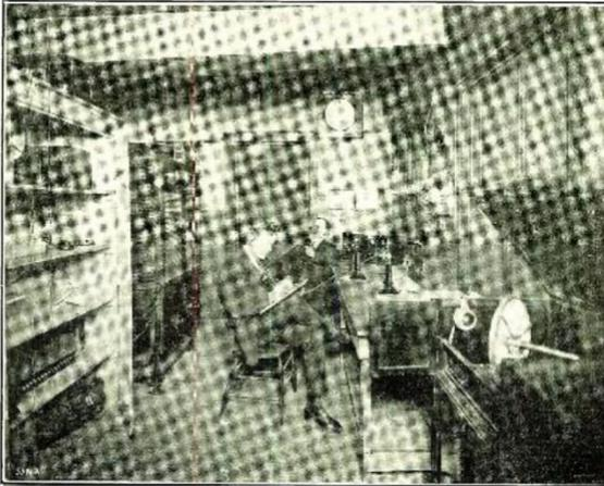
Inside view of the radio-telephone station of the Chicago Opera House. The voice and music are picked up on the stage by several microphones connected to this set and radiated over a large area, enabling anyone with a receiving set to hear the whole performance.
