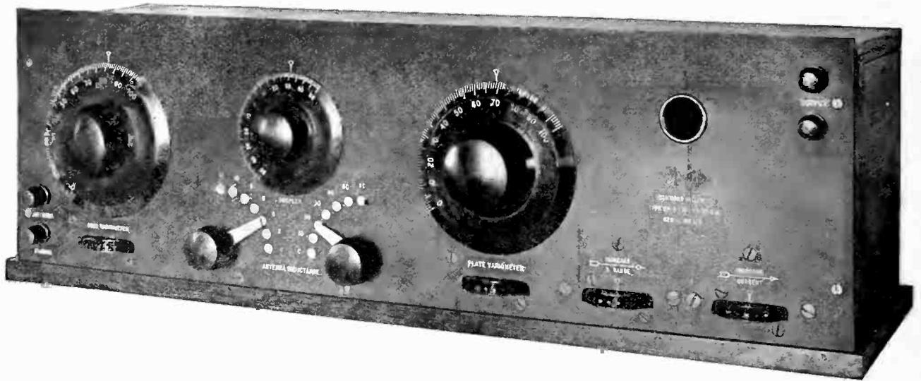
This is a very popular receiving set, covering a wave length range of 150 to 1,000 meters. The set itself is entirely mounted on a single Bakelite supporting panel and is encased by an attractively finished oak box having a hinged cover
