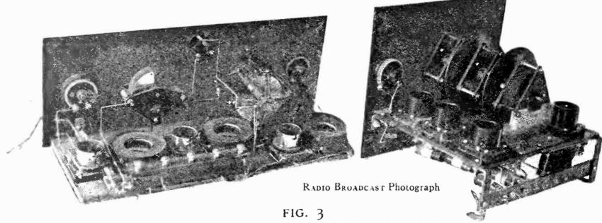
Type of "tandem circuit" sets experimented with in the R. B. Lab. Three circuits and one dial is considerably more difficult than the two control arrangement
