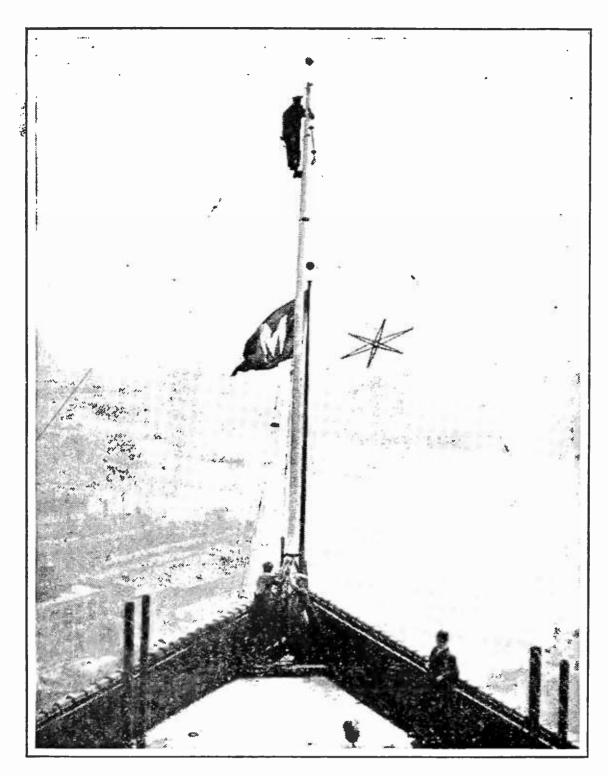
INSTALLING A NEW ANTENNA FOR STATION WCG The New York coastal radio telegraph station of the Independent Wireless Telegraph Company. Many ships in the transatlantic and coastwise service communicate with this station, sending and receiving weather information and commercial messages. This station has a power of  $3\frac{1}{2}$  kw. and will use wavelengths of 600, 706, and 2100 to 2400 meters
