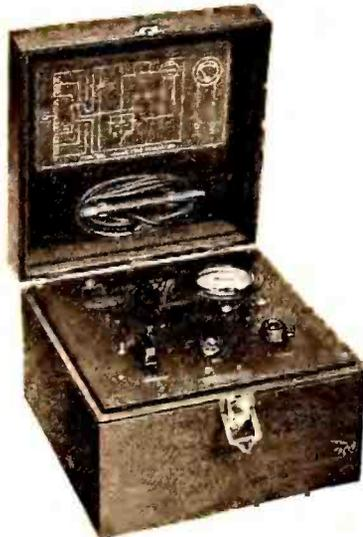
To the service man who prides himself on thoroughness a portable source of radio-frequency signals is indispensable. The aligning of tandem controlled condensers, the neutralizing of receiver or the tuning of the intermediate-frequency amplifier in a superheterodyne receiver all require a dependable test signal.
