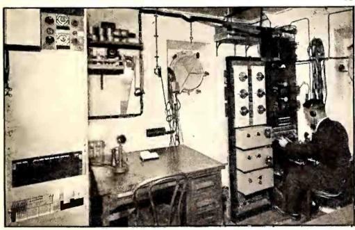
The inauguration of two-way ship-to-shore telephone service on the S.S. Leviathan makes it possible for any passenger to transact business or talk with friends by telephone while crossing the Atlantic. This picture shows the radio telephone equipment on the Leviathan. To the right is the receiving apparatus where voices from shore telephones are received by radio from the Deal (N. J.) station.
