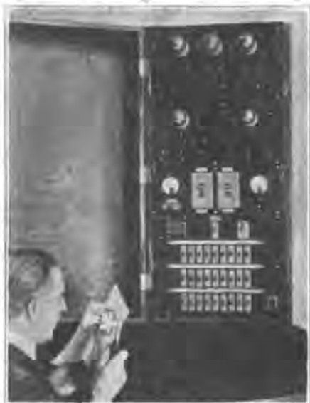
Talking to the pupils of 25 classrooms at one time by means of a Magnavox Telemegaphone installation equipped with radio hook-up.
