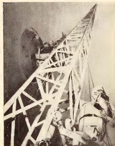
WBAP-TV Fort Worth moved a step nearer to network telecasting with the installation July 14 of a 200-ft. portable microwave test tower. AT&T Engineer A. T. Chinn is shown making a last-minute check. Readings obtained by AT&T will determine height, size and design of a permanent tower for WBAP-TV's network link. WBAP-TV plans a $250,000 Fort Worth terminus of the transcontinental AT&T network.
